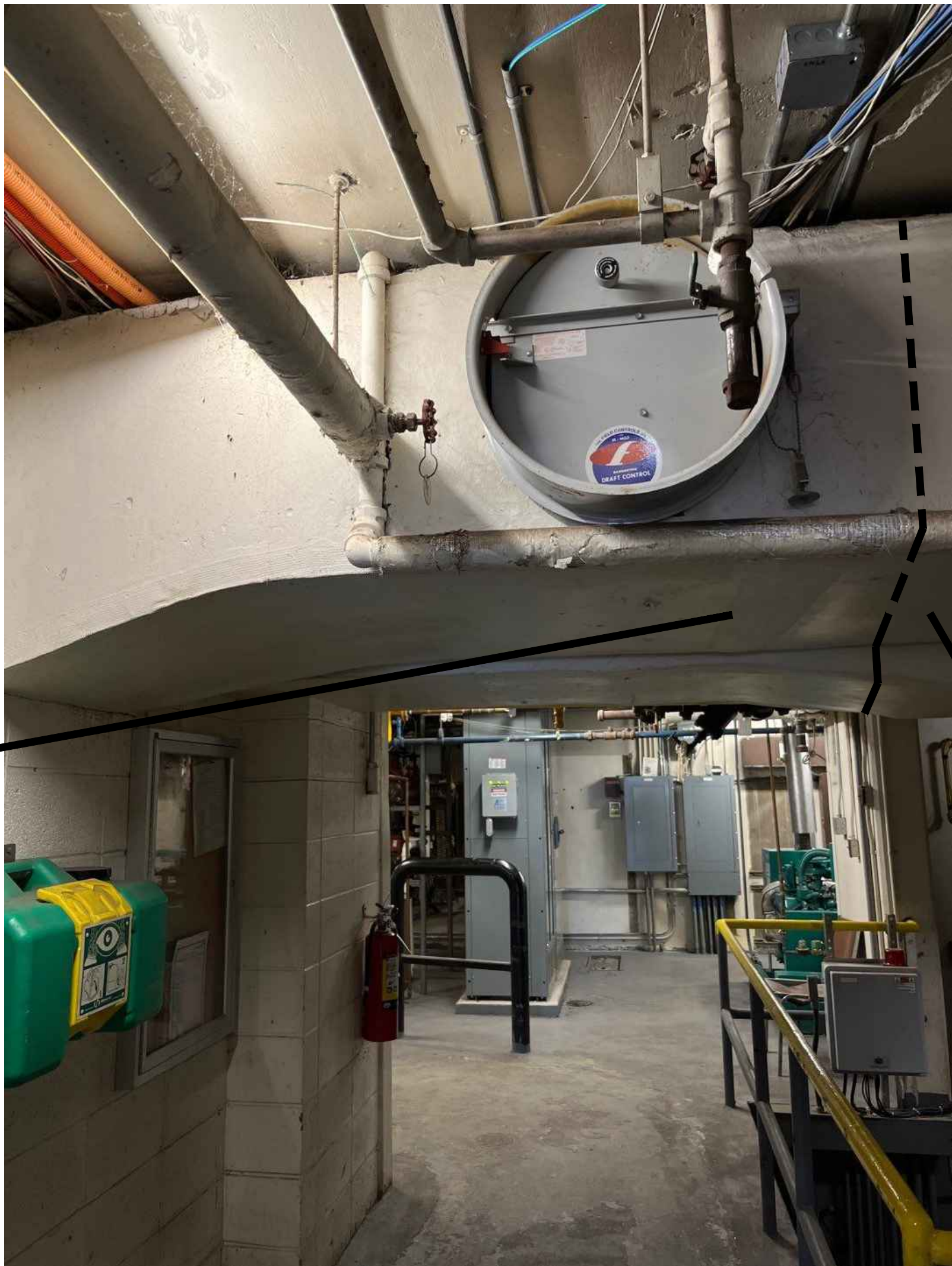
APPROXIMATE LIMIT OF BREECHING TO BE REMOVED DURING PHASES I AND II, TO BE CONFIRMED WITH OWNER
